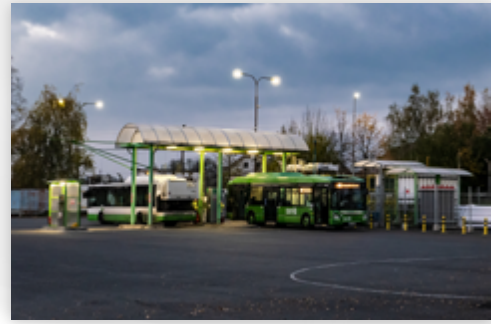
CNG Fueling Construction
